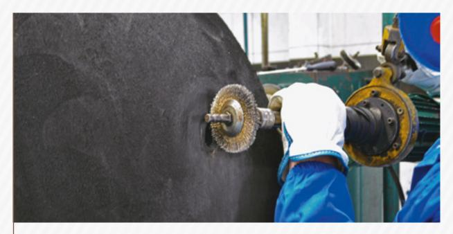
Remove the burnt rubber from the skived area with the aid of a steel brush (for tyres/tires with steel belts) or tungsten ball pin.
