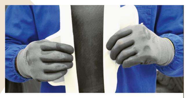
Remove the protective film from the patch from the hump to the edges, leaving room to ensure the repair and preventing contamination of the base.
