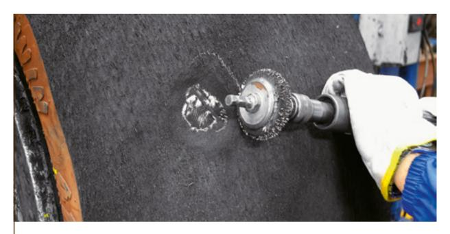
Skive the damage in a concave way, removing the loose rubber, preparing the damage so to avoid straight or too open angles that hamper the filling's anchorage.
